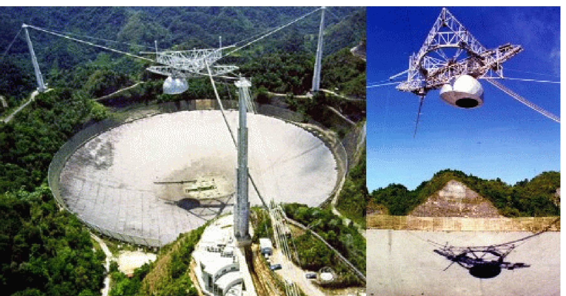
Figure 1. A photo of the NAIC 305 meter telescope at Arecibo. The inset at right shows the details of the "carriage house" structure. The feed used by this project is the line feed extending downward from the carriage house. (Photos courtesy of NAIC-Arecibo Observatory, a facility of the NSF)
